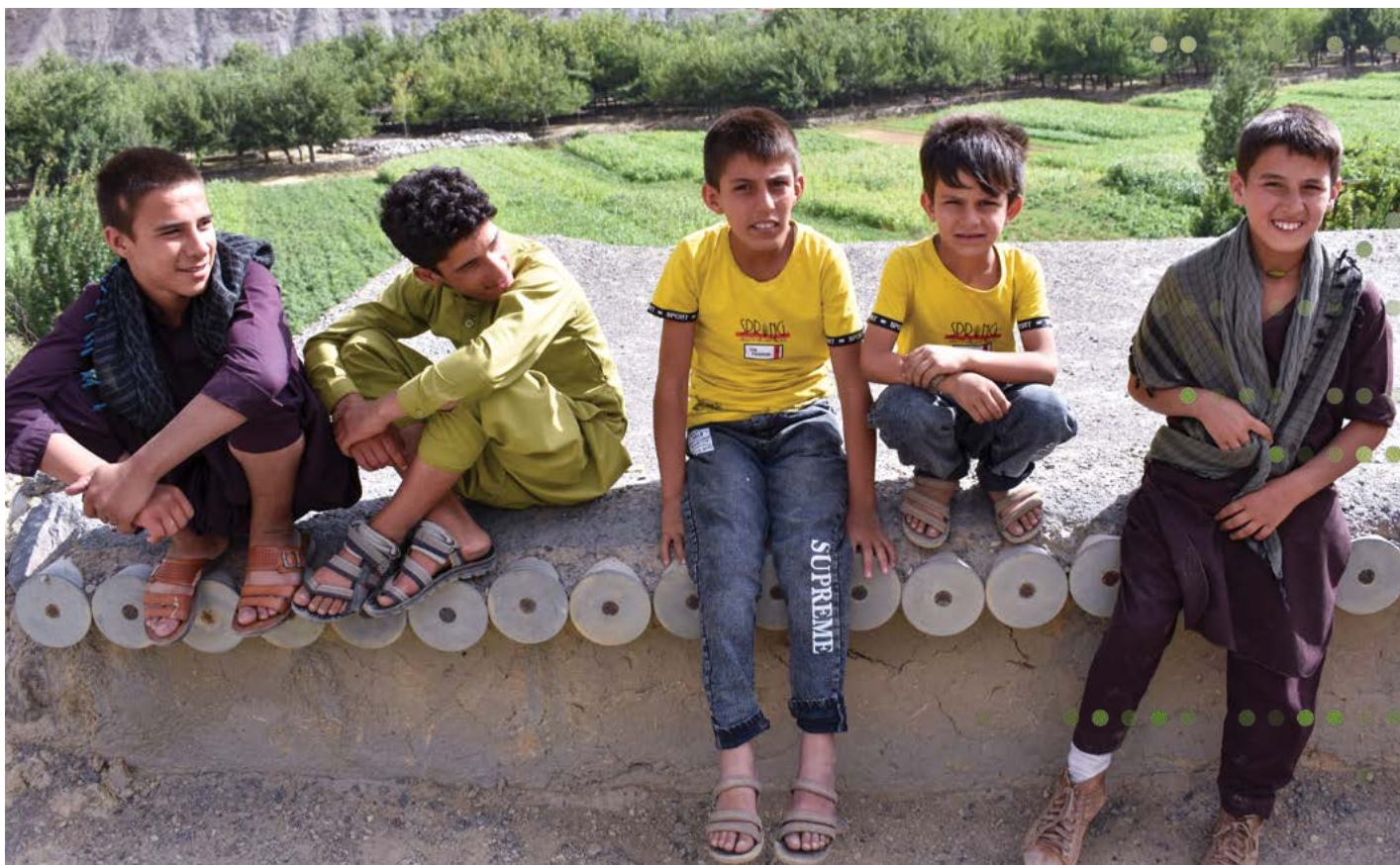
BUILDING SOMETHING NEW: Levine took this photo in Sangana, Afghanistan. The supports for the roof the children are sitting on are old Soviet artillery shells with the explosives removed. They're commonly used as building materials in this area.
