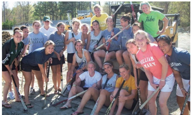
Members of the William and Mary field hockey team help renovate the turf at Busch Field, home to the team since 1989. The original surface was torn out in April.
